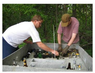
**step 7: Leveling and Laying**I poured buckets full of thick mud into the void above the bottles, and screeded the whole mess with a big 2x4.
