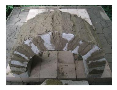
step 9: CastlingWe built a sandcastle the shape of the oven void. Negative space!We'll dig the sand out through the door when the oven is completely built and dried.
